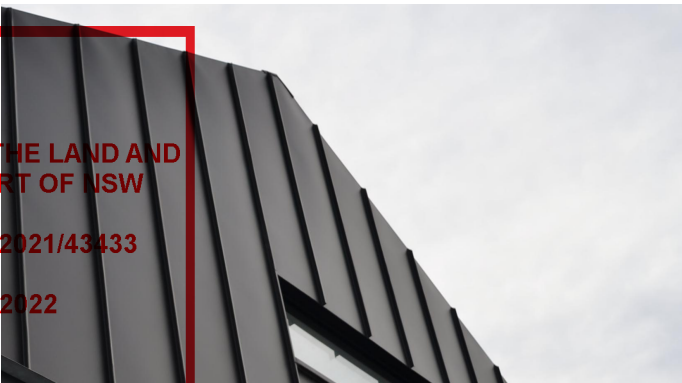
MC1 - ALUMINIUM ROOF CLADDING - DARK COLOUR
